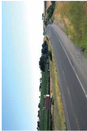
State Highway: Agriculture & Residential Limited-access road with gravel shoulder.
